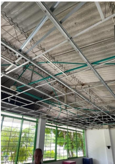
Desmante cielo falso panel yeso
