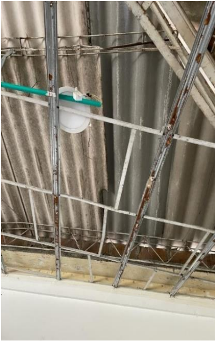
Desmonte cielo falso panel yeso
